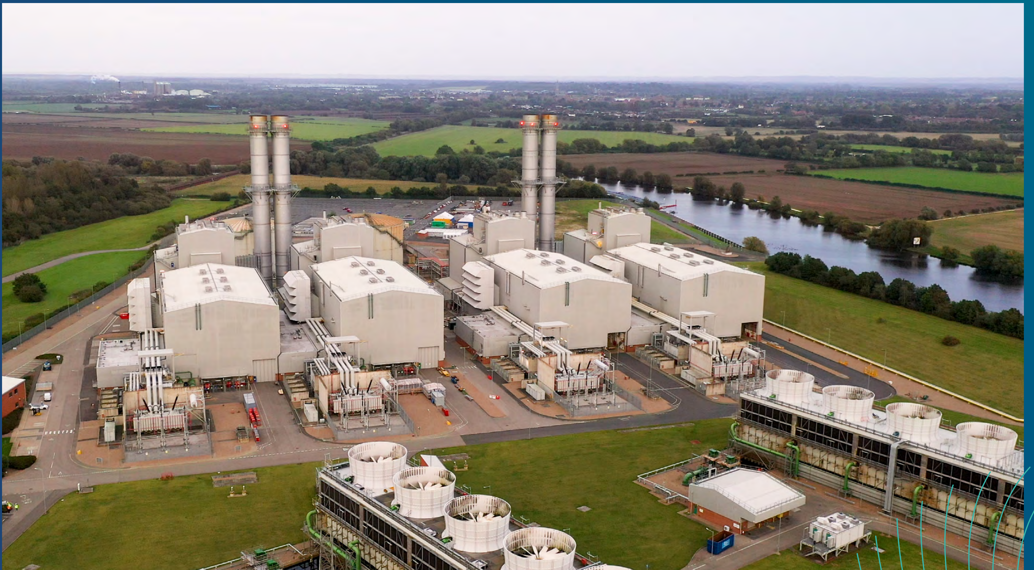
Staythorpe Power Station
