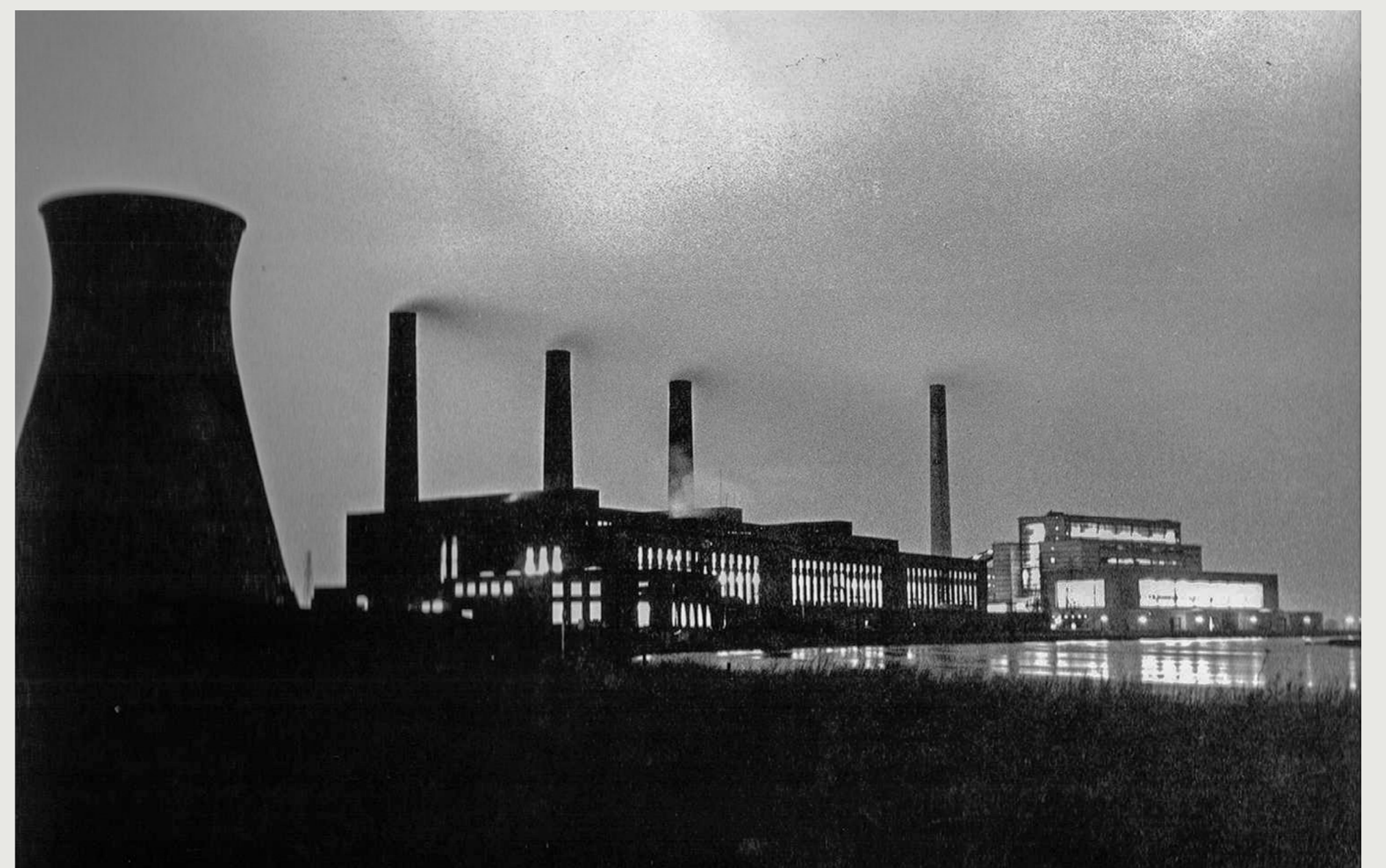
Staythorpe A & B Power Stations
